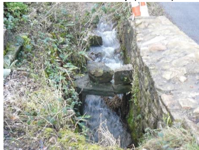
10. Culvert collapse (since repaired) near to the quarry entrance.
