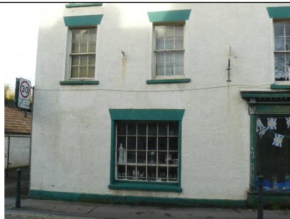
GO10 , sash windows, display window beginning to bow, poor condition.
